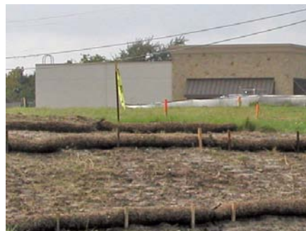
Ribbon to slow water flow on long slopes
