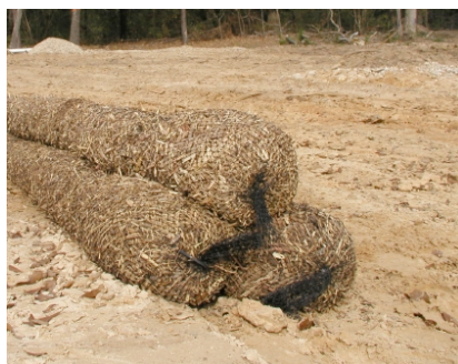
Pyramid for large field sheet flows
